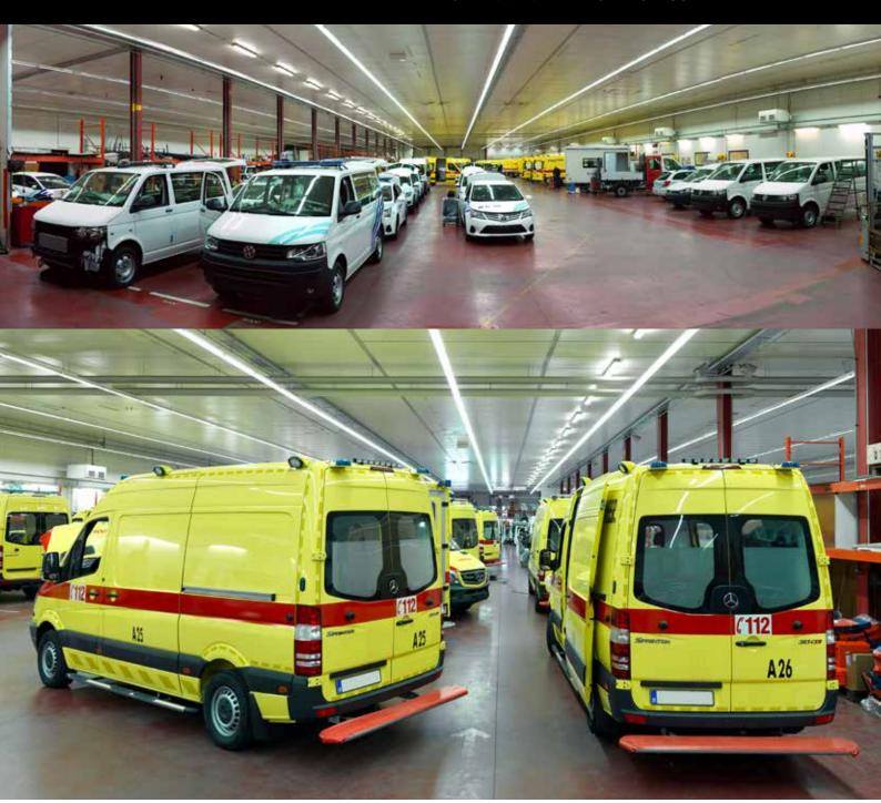
These exacting performance requirements were ably met with the combination of luminaires from the Sylvania Range from Havells Sylvania. The Sylvania FTS was specified supplemented with Sylproof Superia LED waterproof luminaires on the walls. In total, 636 FTS modules were suspended in the hall and 22 Sylproof Superia LED waterproof luminaires were installed by electrical engineer, Nizet SA.
